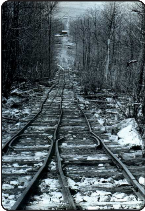
Photo showing the “tracks” going down the slope around 1900, perhaps still in the building stages.
